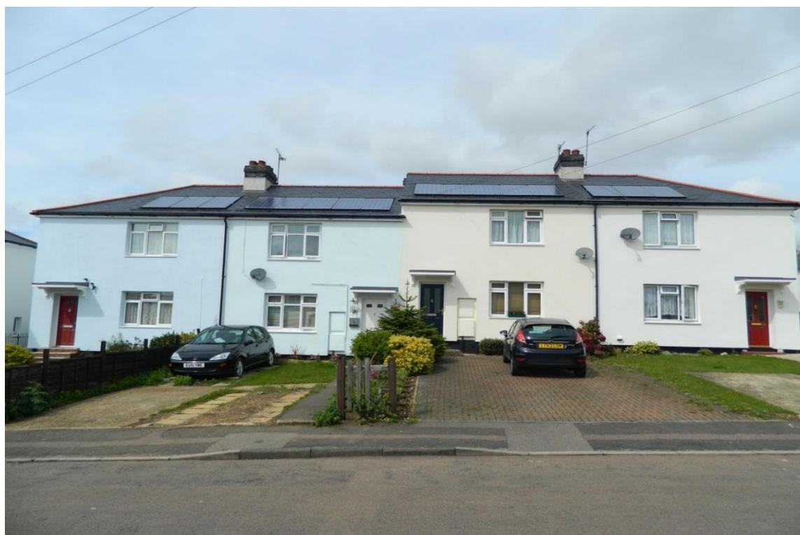
The upgrade of the block of **20 flats** in Longlands, in the image below, included EWI, solar PV and new double glazed windows to all properties and the communal areas, as well as providing six additional flats on the roof for social rent.
